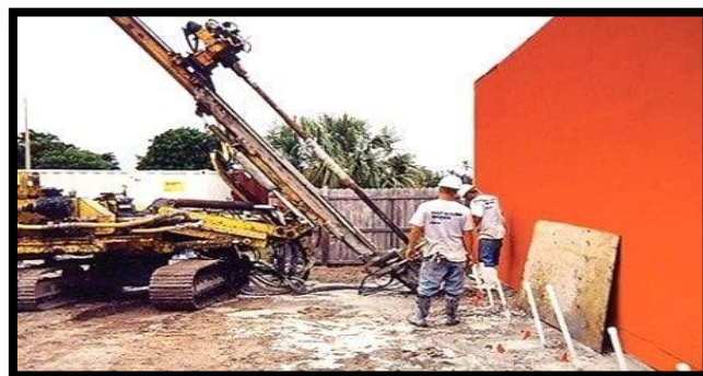
Fig.5.5.1. – chemical grouting
